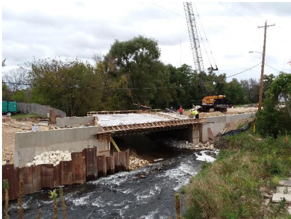
Bridge deck covered for seven-day curing period
