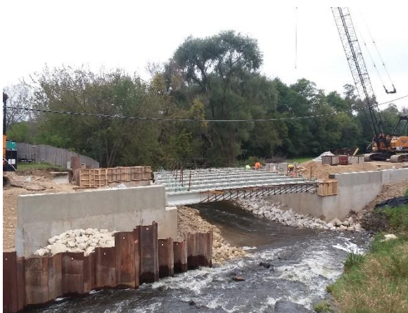
Bridge girders were placed on Sat. 9-22-18
