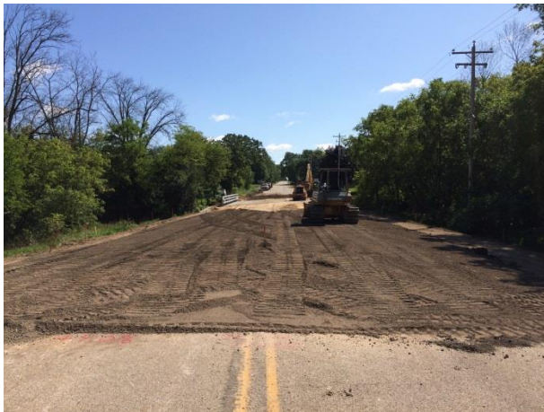
Approach Reconstruction (Photo Looking East)
