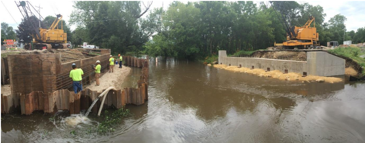
Photo Looking South - Constructing Forms and Installing Reinforcing Steel for East Abutment (7-10-17)
