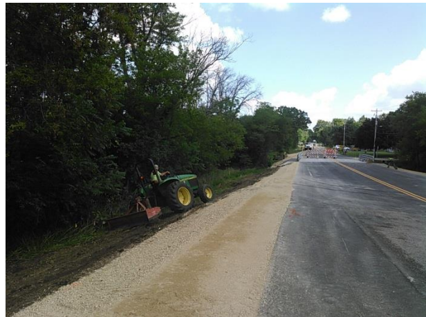
Asphalt Paving Complete – Landscape Restoration Underway
