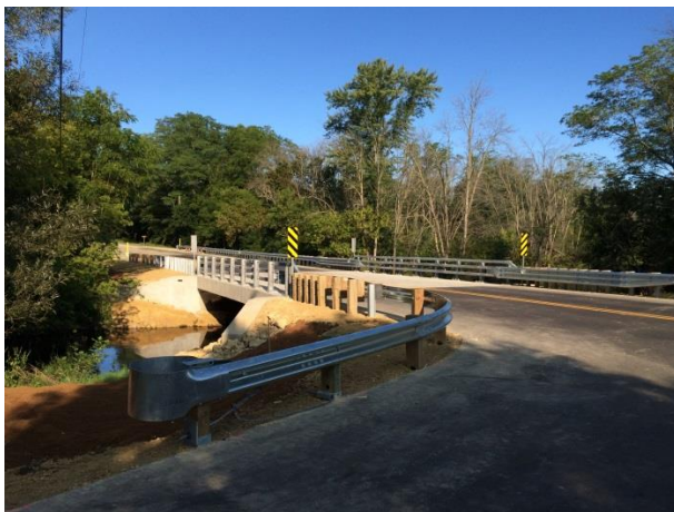
Guard Rail Installed
